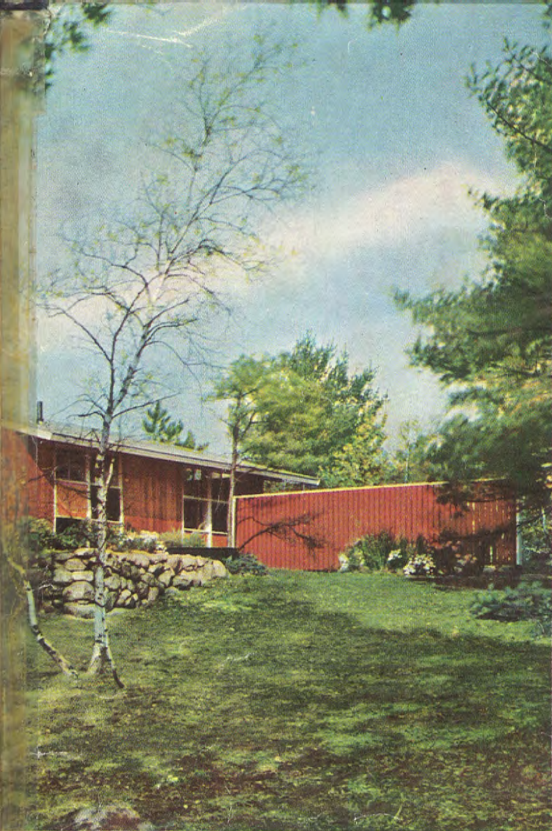
Picture on the cover shows this two-story end where concrete foundation walls enclose daylight living space in "basement." Vibrant panels and glass in four-foot widths are part of many ideas in house of prefabricated parts
