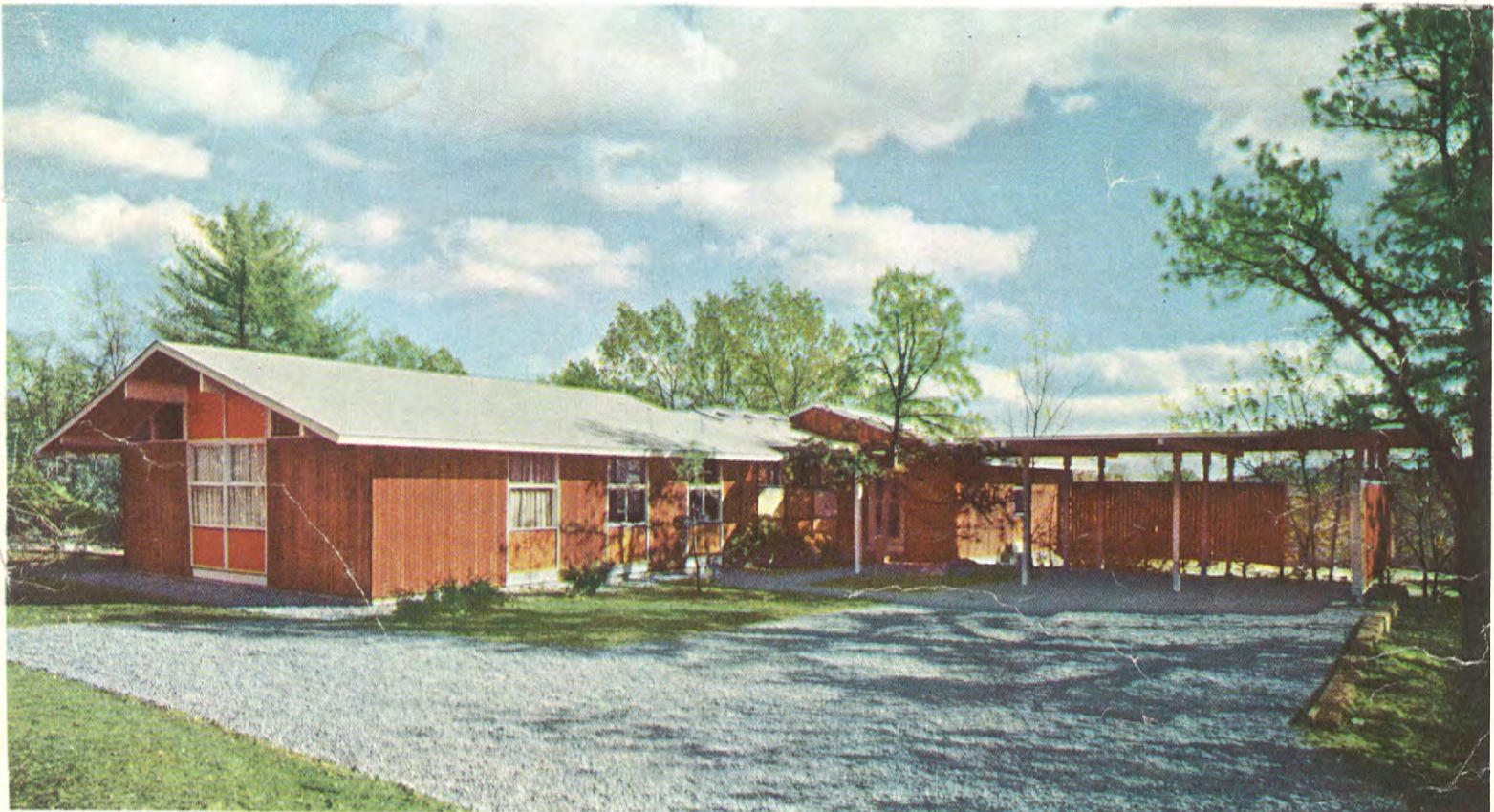
Like house itself, double carport is exciting in its simplicity. Its outside walls are merely framed vertical board fence fastened to carport posts. Panels, used
